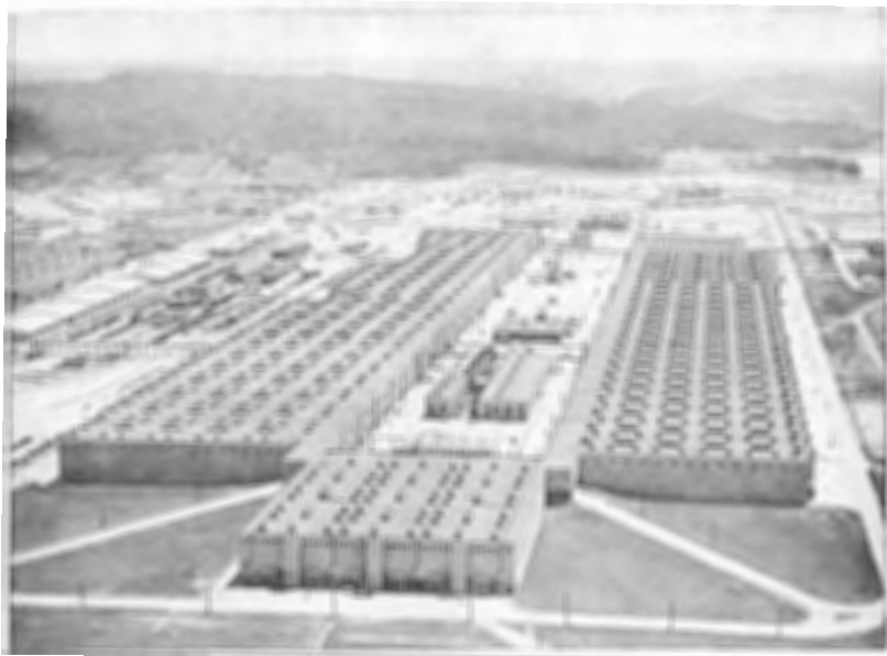
FIG. 20-4. Diffusion plant of the Clinton Works (now Atomic Energy Commission) at Oak Ridge, Tenn., for the separation of uranium isotopes.
